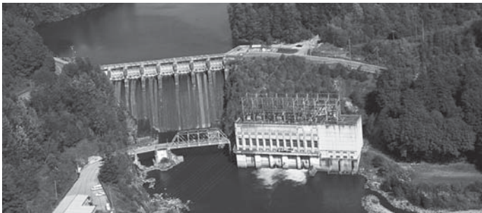
Ruskin Dam and Powerhouse, BC. (Photo courtesy of BC Hydro.)
